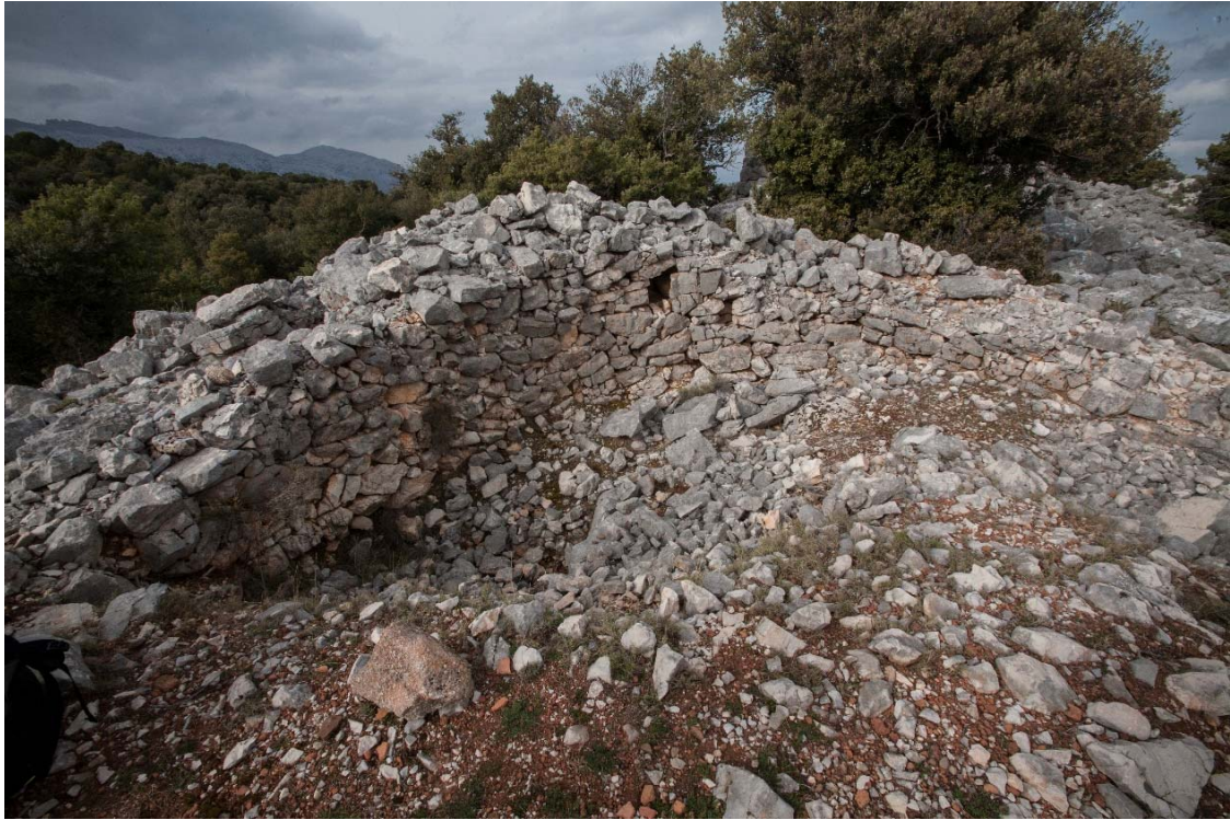
Fig. 8. Campu Doinanicoro. Struttura "a muraglia". Undetermined structure with large walls.
