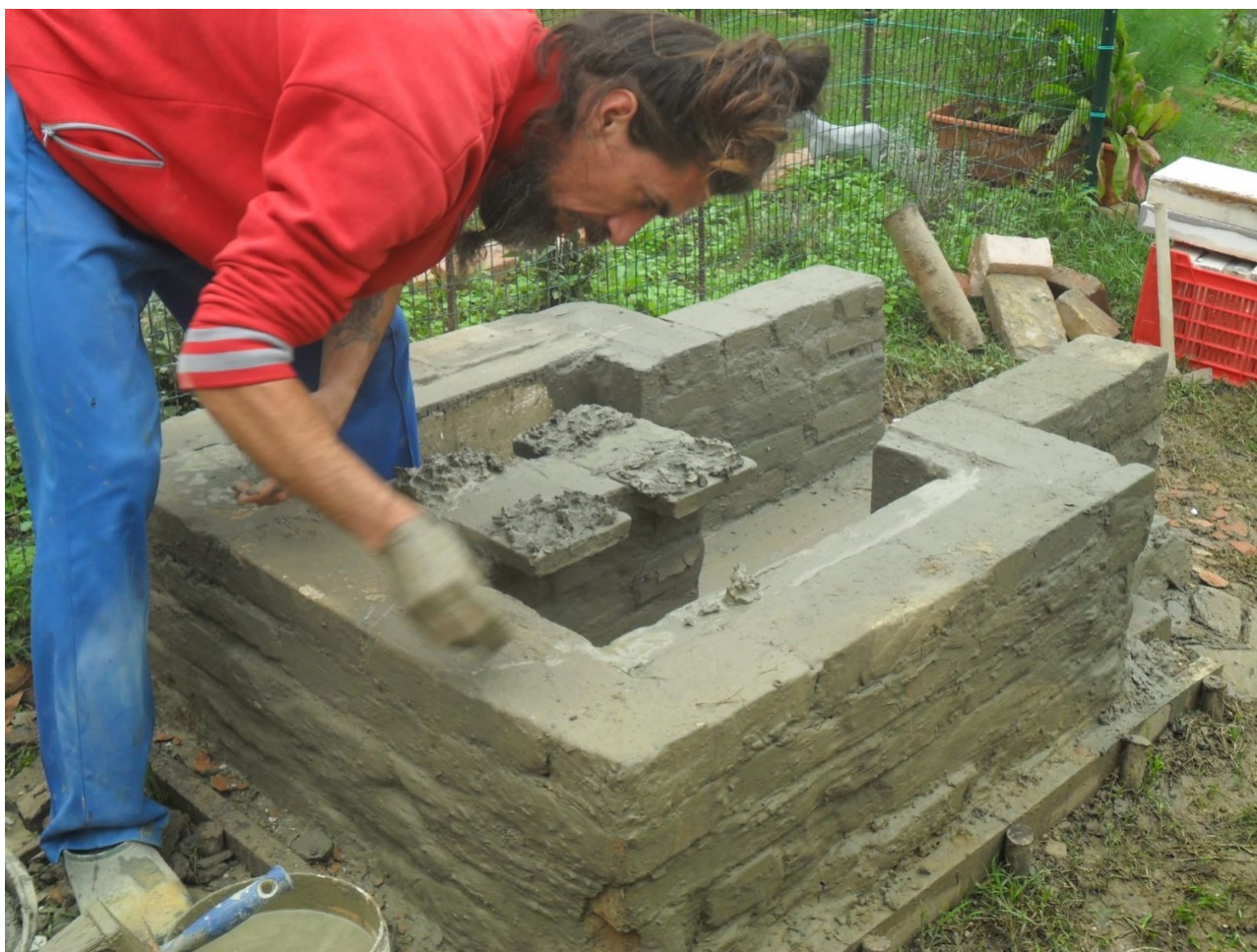
Fig.5. Fornace in mattoni ad alte temperature. Kiln made of bricks for high temperature.
